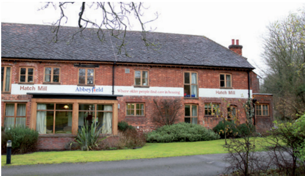
Hatch Mill Nursing Home - Farnham Surrey
