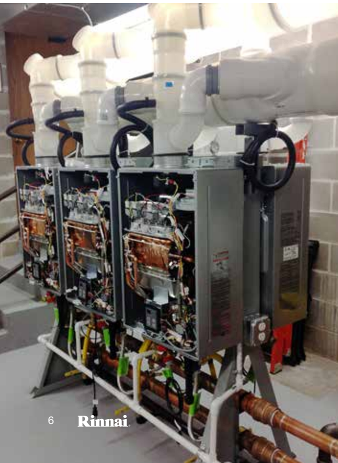
County Courthouse: TRS06i with Common Vent (1.2M BTU)
