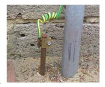
The mechanical installation must ensure that the AP is grounded to earth ground to dissipate static electric charge that may develop due to wind. In Step 3 on page 3, you secured a grounding wire to the AP.
