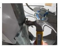
Using a hammer, bend and flatten the two tabs on the buckle, so that they hold the flattened strap end in place.
