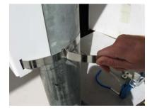
Using the Band-It tool, place the tool onto the strap.
