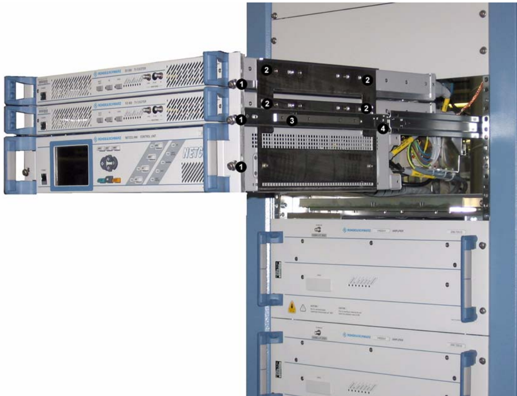
Fig. 16 Removing the exciter from the transmitter rack
