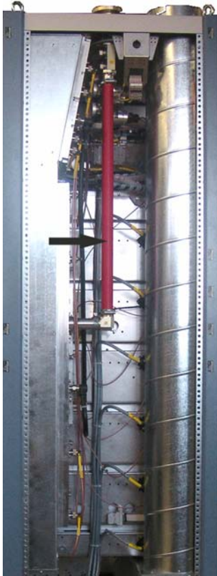
Fig. 19 Removing the harmonics filter
