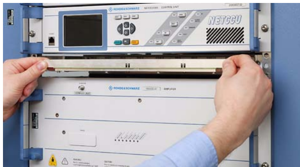
Fig. 15 Removal of rack controller from transmitter rack: removing rack controller
