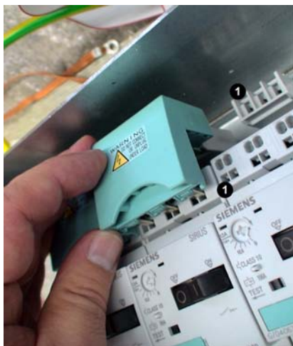
Fig. 6 Installing the motor protection switch
