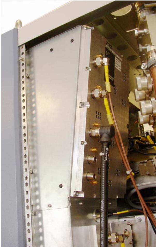
Fig. 18 Removing the absorber
