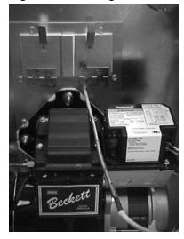
Check the initial draft setting as the furnace warms up. The draft may be measured at the test port. The breech draft should be approximately - 0.05" w.c. to obtain an over fire draft reading of - 0.02 inches w.c.
