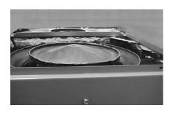
Heat Exchanger Support Screw In the upflow position, the heat exchanger support screw shown in picture may be removed. This may be preferable if the furnace rear panel will be inaccessible after installation. The screw must be removed if the heat exchanger must be removed from the cabinet. Do not remove this screw if installing furnace in a horizontal position.
