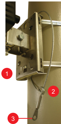
Figure 28. Secured safety cable
