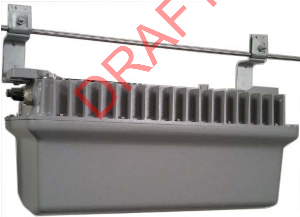
Figure 1. Typical T504 mounted on a strand
