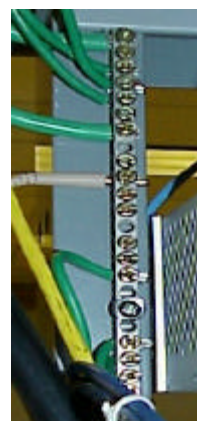
Detail of Equipment Rack Ground Block
