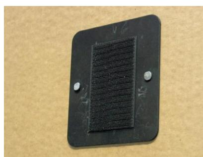
3. If necessary, prepare the installation of the SID and RADs by installing the plate and/or velcro kit.
