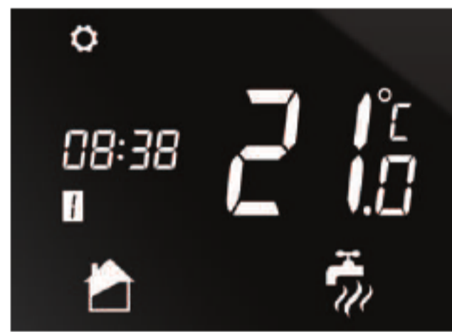
Central heating and hot water
