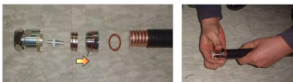
Figure C.5 Assembling the Din type-male (1/2 in. Feeder Line) Connector (1)
