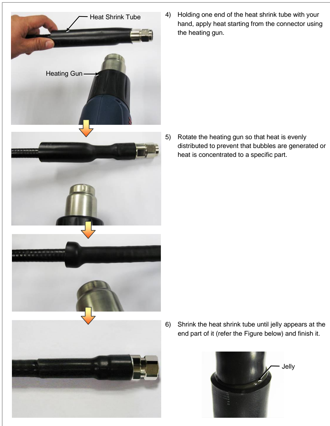
Figure C.9 Shrinking the Heat Shrink Tube_Feeder Line (2)
