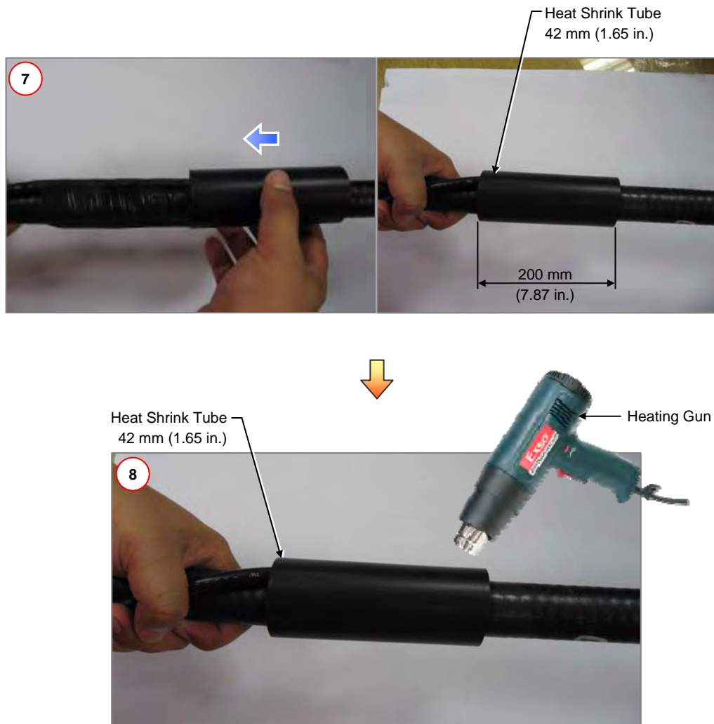
Figure B.3 Feeder Cable Grounding (3)
