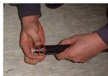
Figure C.5 Assembling the Din type-male (1/2 in. Feeder Line) Connector (1)
