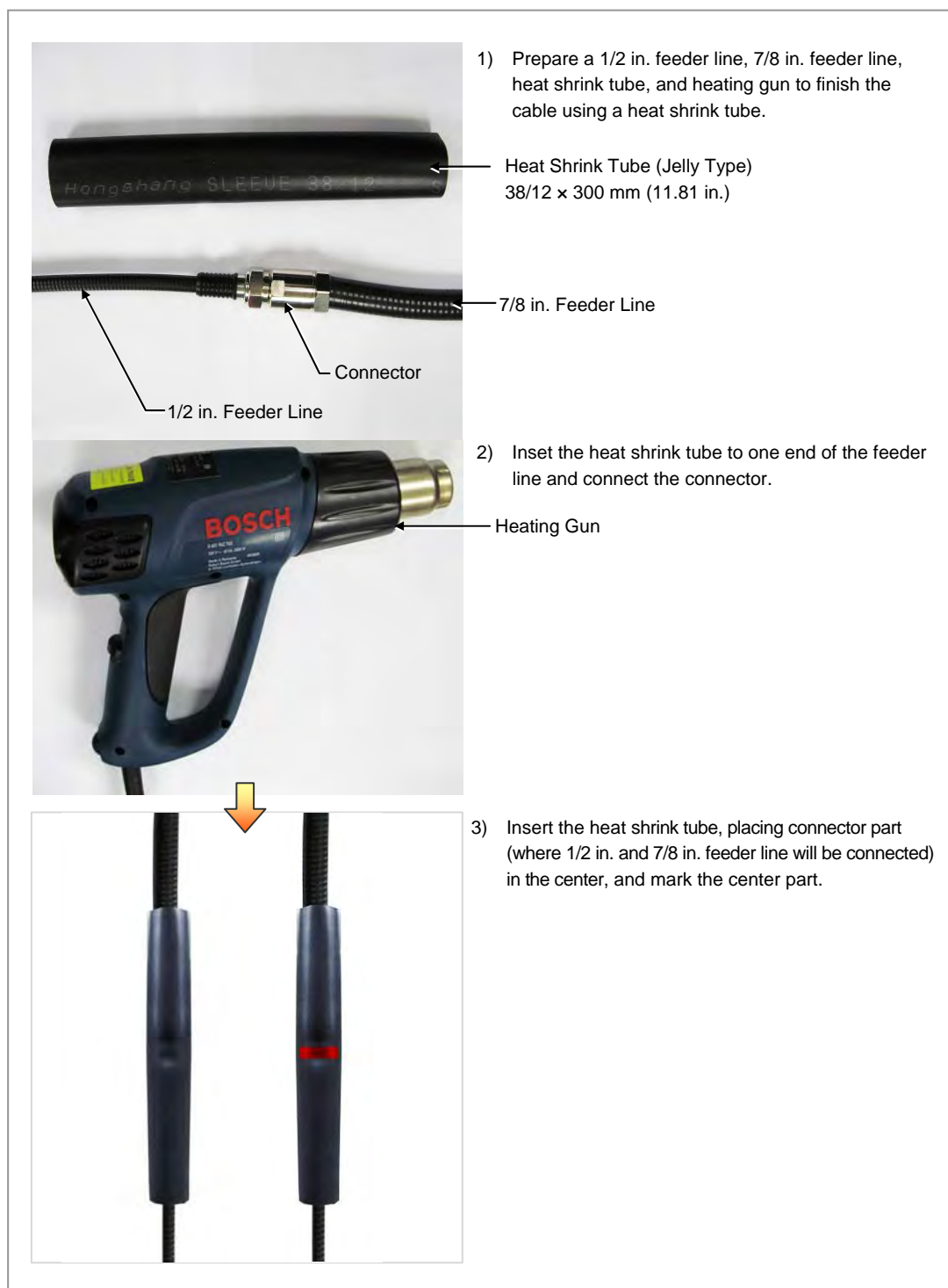
Figure C.10 Shrinking the Heat Shrink Tube Connection between Connectors (1)
