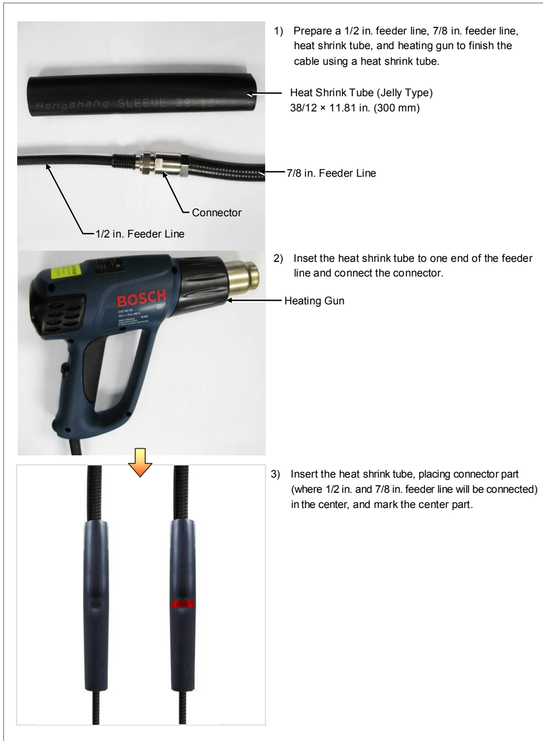
Figure C.17 Shrinking the Heat Shrink Tube_Connection between Connectors (1)
