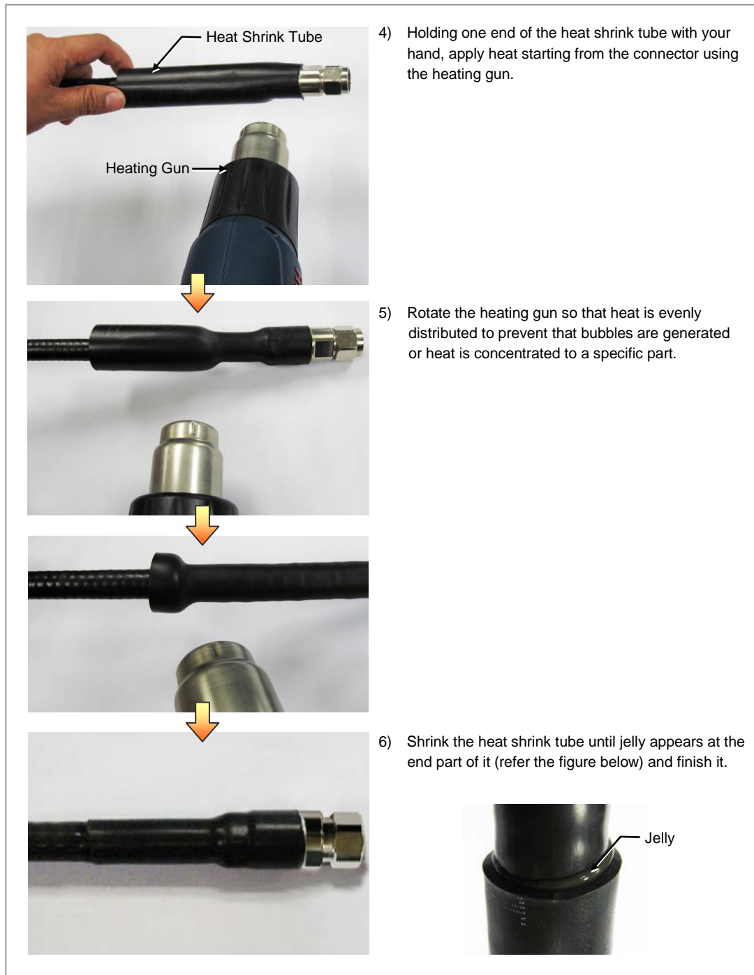
Figure C.16 Shrinking the Heat Shrink Tube-Feeder line (2)
