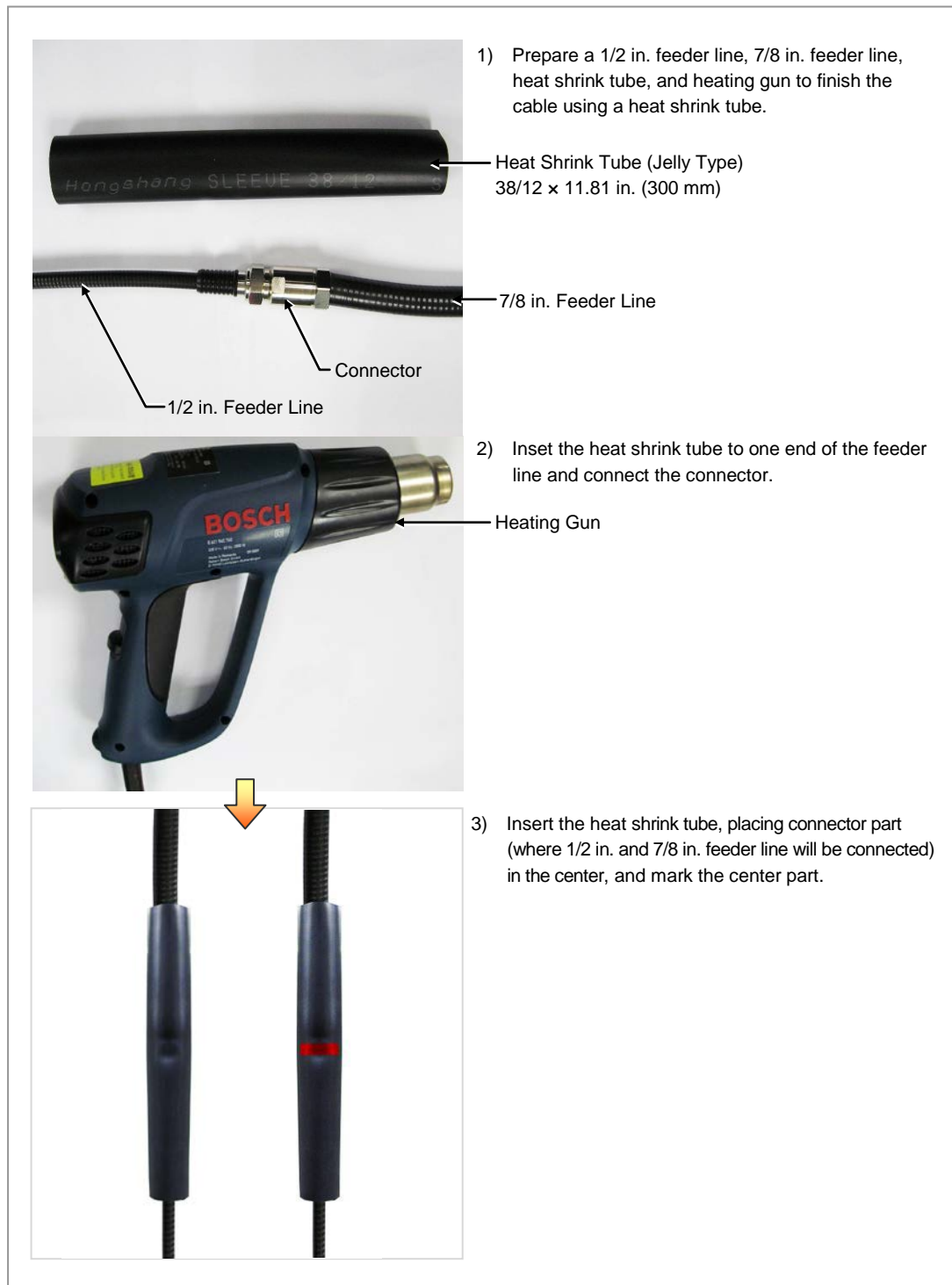
Figure C.17 Shrinking the Heat Shrink Tube-Connector (1)
