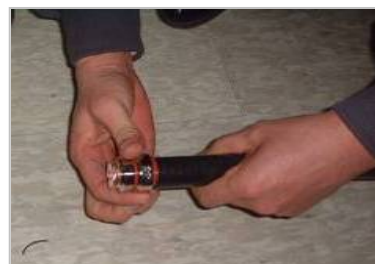
Figure C.12 Assembling the Din type-male Connector (1/2 in. Feeder Line) (1)
