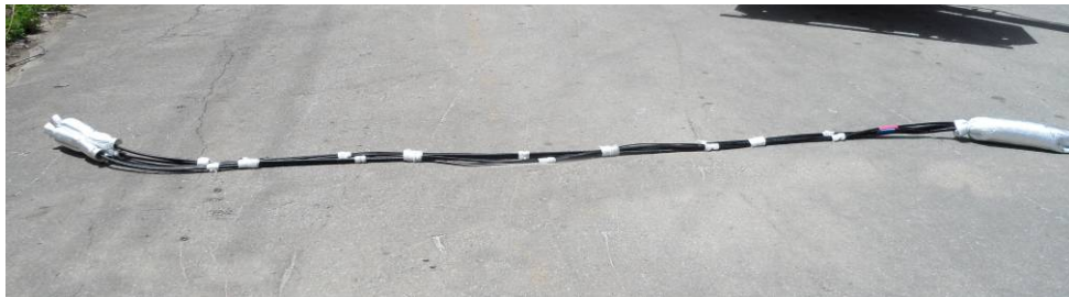
Figure 2.14 Installing Hybrid cable (2)
