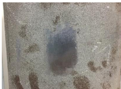
Figure 5 Pipe preparation prior to ultrasound sensor installation (from HotSense® instructions)
