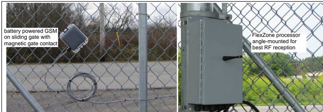
Figure 7 Angle-mounted FlexZone processor and gate sensor module
