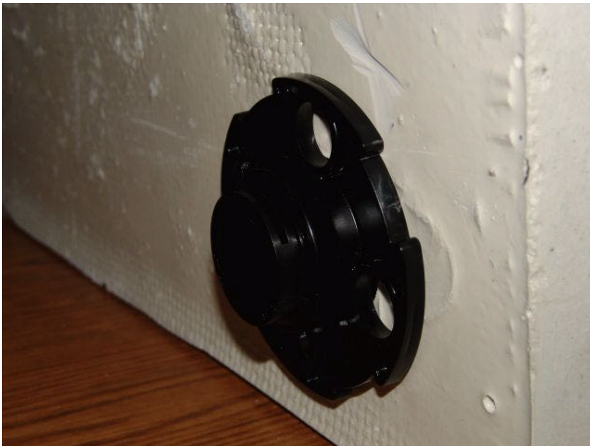
Securing the Pit Lid Housing to the Pit Lid
