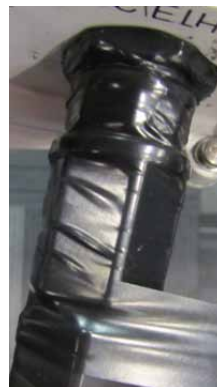
Figure 4.7. Wrapping the Connector with Electrical Tape
