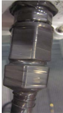
Figure 3.17. Wrapping the Cable with Rubber-splicing or Self-amalgamating Tape
