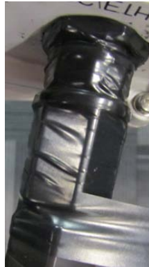
Figure 3.18. Wrapping the Connector with Electrical Tape
