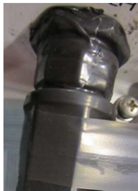
Figure 3.16. Wrapping the Connector with Rubber-splicing or Self-amalgamating Tape
