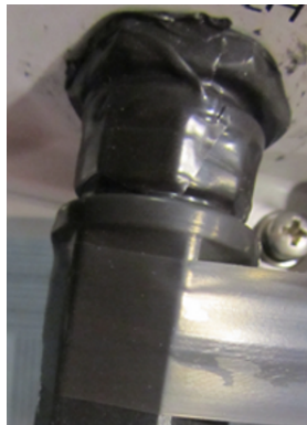
Figure 19: Wrapping the Connector with Rubber-splicing or Self-amalgamating Tape
