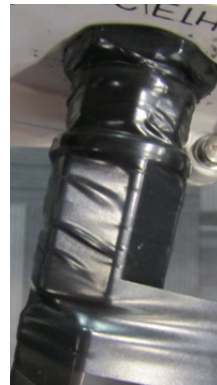
Figure 21: Wrapping the Connector with Electrical Tape
