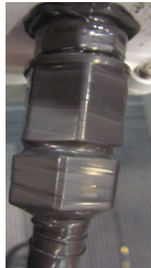
Figure 20: Wrapping the Cable with Rubber-splicing or Self-amalgamating Tape
