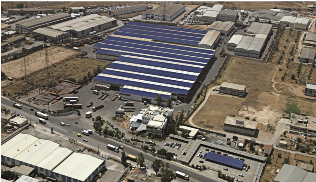
A SINVERT PVS2000 is used for the Aspropyrgos 2 MW roof system erected in Greece in 2011 for Big Solar
