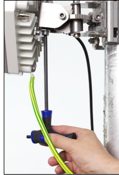
(b) Vertical (elevation) adjustment screw
