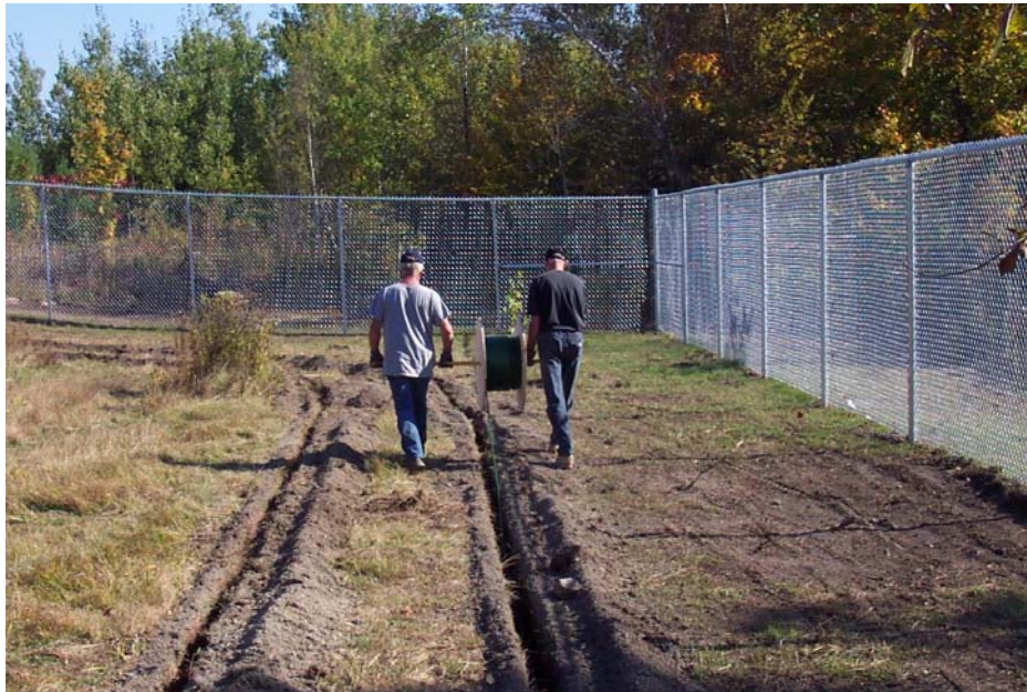
Figure 5.8 Spooling-off a Sensor Cable Assembly
