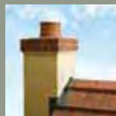
Brick/Stone Chimney (Class 1) 1
