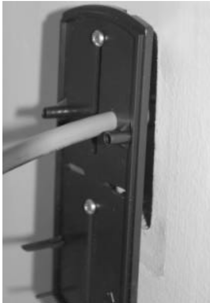
Figure 6> Installing back plate to the wall
