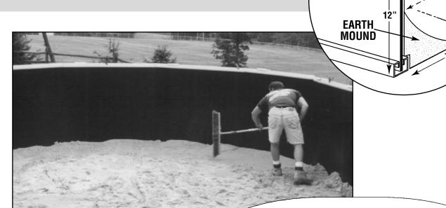
Build earth mound on top of wall guard using screened damp earth or pre-washed sand.
