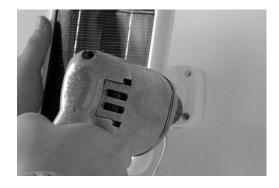
5) Drill holes with an appropriate drill bit and insert plastic anchors into stucco, concrete or brick.
