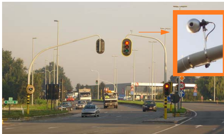
Figure 1: TrafiCam® installed at an intersection
