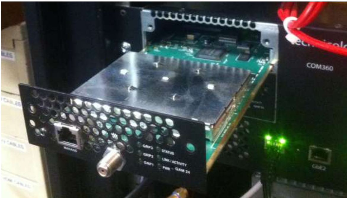
Figure 8 – QAM6 board being installed in COM360
