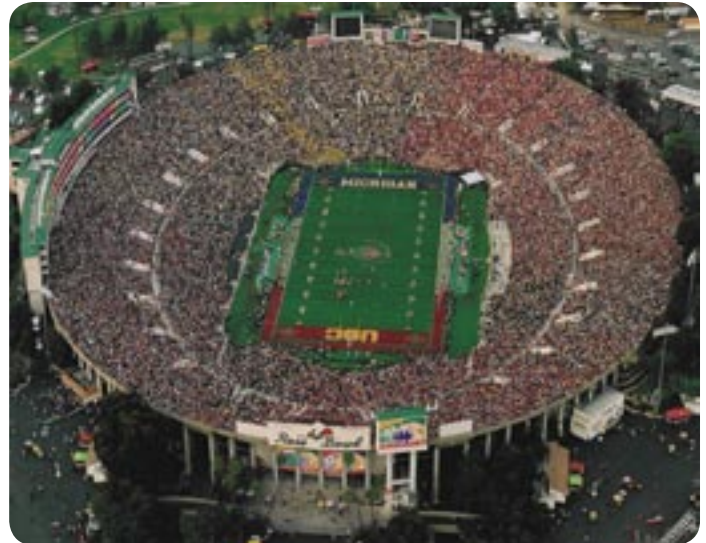
The Sentinel central control system helps keep the Rose Bowl looking good.
