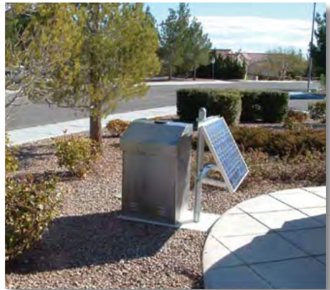
Solar-powered Controller Retrofit or areas like highway mediums where standard 120 VAC can't be run to.
