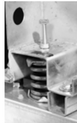
Figure 3. Spring Isolation
