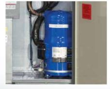
**Digital scroll compressors** — by operating at constant speed and digitally controlling position of the orbital scroll in relation to the fixed scroll, very precise capacity matching at part load conditions can be achieved.
