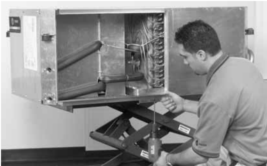
Figure 52. Install top/bottom filter rack
