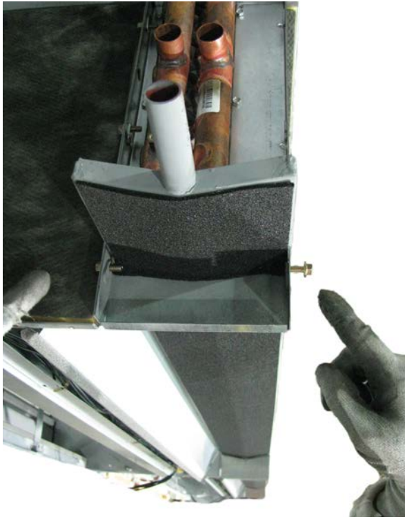
Figure 58. Removal of screws holding drain pan in place.
