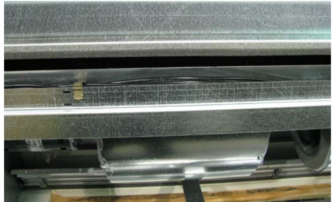
Figure 59. Tie wires from the cable chase out of the way
