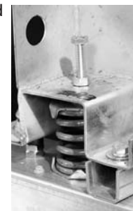
Figure 5. Spring isolation
