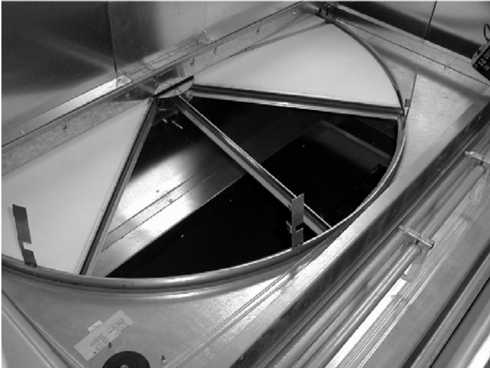
Figure 107. Segment Removal
