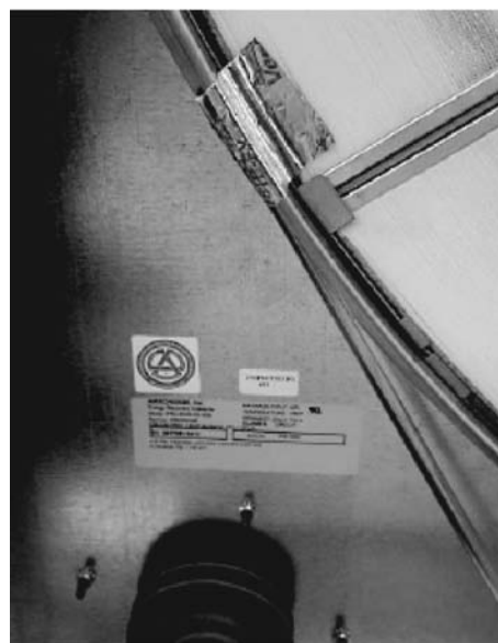
Figure 110. Link belt installation
