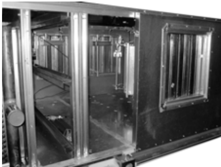
Figure 51. Outdoor economizer section
