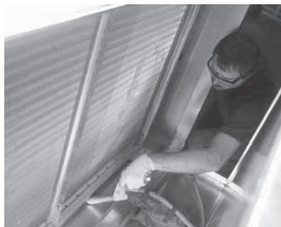
Figure 40. Extended drain pans for easy cleaning
