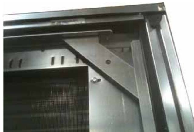
Figure 21. Coil structural gusset
