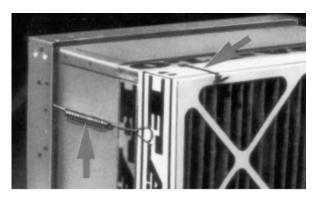
Most filters in custom units are installed in unitary sheet metal frames. If unit is provided with side access rack, do the following for installation:
