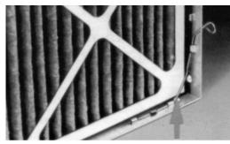
Figure 46. Bag filter show with C-70 fastener
