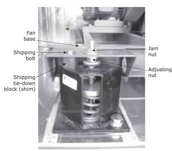
Isolators are selected for distribution of equipment weight, but may not all compress the same. This procedure assumes the base surface is level. Isolators are not intended to be leveling devices.
