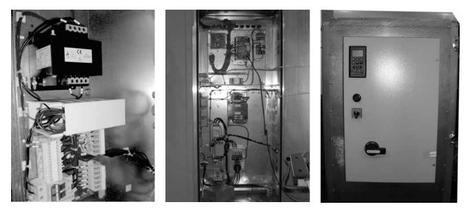
All units with starters or variable-frequency drives (VFDs) that have direct-digital controllers (DDCs) are provided with line voltage to 120 Vac power transformers (see Figure 67) with power 120 Vac to 24 Vac control transformers (see Figure 68). Figure 69 shows a typical VFD power box.
