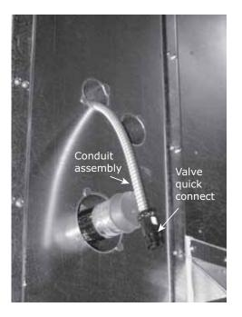
Figure 70. Valve jack wiring details
