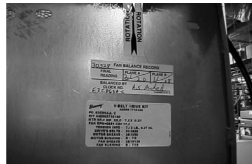
Figure 47. Location of fan belt label on fan scroll (top) and belt tensioning with fan adjustment points (bottom)
