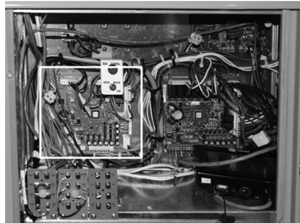
Figure 13. Precedent™ E Cabinet - RTOM board
