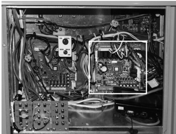
Figure 11. Precedent™ B Cabinet - RTRM board
