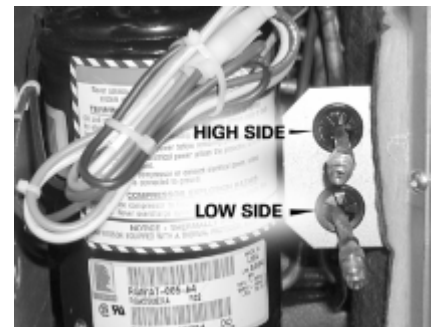
Figure 8: Schrader connections
