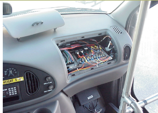
Example of an Auxiliary Electrical Panel on a Ford Van
