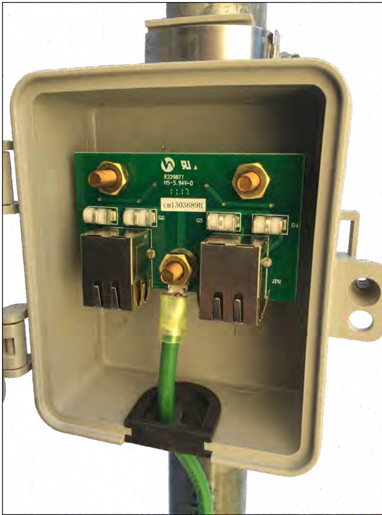
Figure 15: Ground wire installed on surge suppressor
