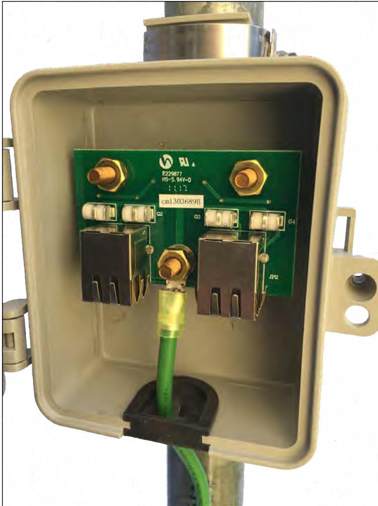
Figure 15: Ground wire installed on surge suppressor
