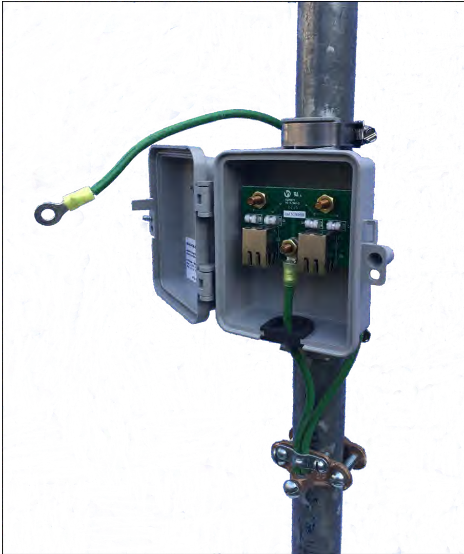
Figure 17: Attach the ground wire
