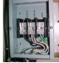
Figure 3-3: AC Input Box Assembly
