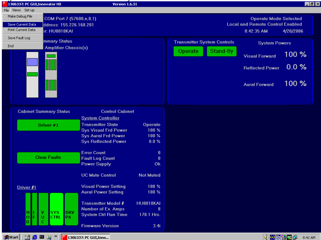
Figure 3-8 Control/Exciter Cabinet System Controller Screen
