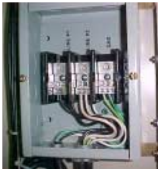
Figure 3-4: AC Input Box Assembly
